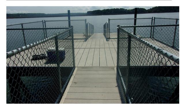
Dock, observed to be in good condition Note metal surfacing, aluminum railings
